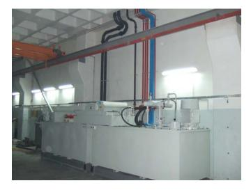
The Main Settling tanks can hold up to approx. 6000 Litres of Neat Oil and is accessible through the removable top plates. Each tank is divided into smaller sections of baffles and both are united via a transfer tube. There is a 37 KW Motor drives a Gear-pump, for the hydraulic circuit
